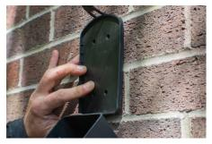
• Now use the 5mm drill bit to make a hole 110mm deep in each of the marked fixing holes
