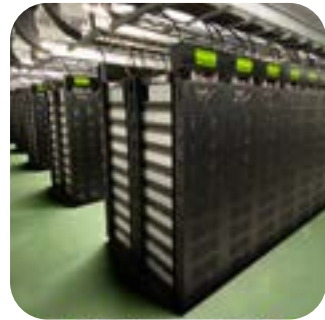
BESS Battery Energy Storage System
